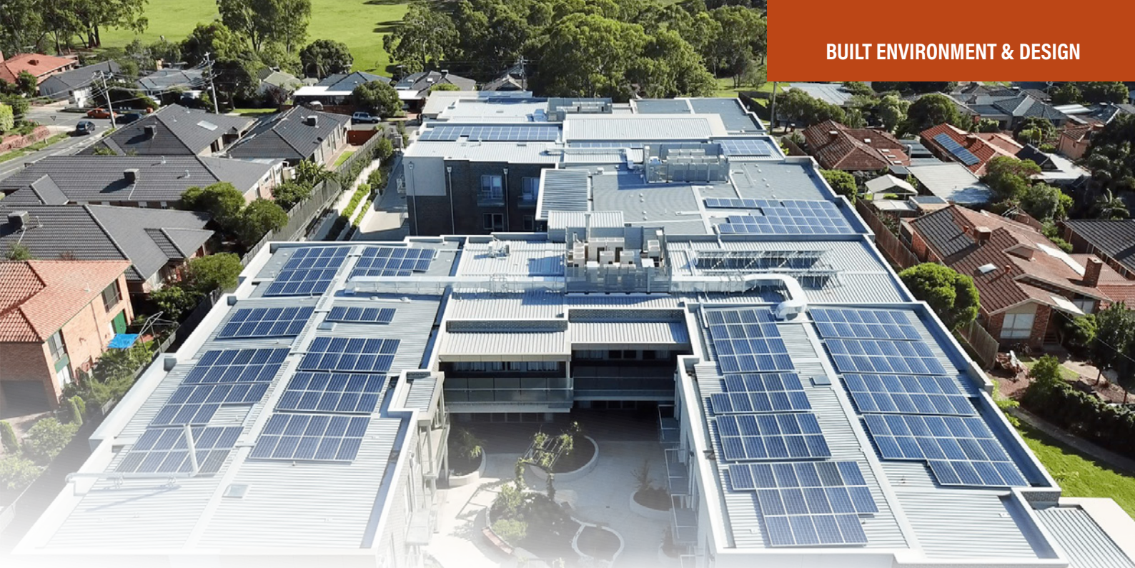
Solar Installation at Trinity Manor Aged Care, Greensborough.
