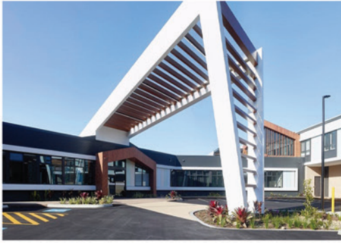
Plumbing, Draining & Gas Maintenance
