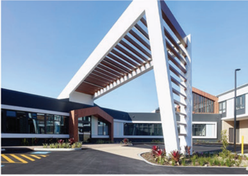
Plumbing, Draining & Gas Maintenance
