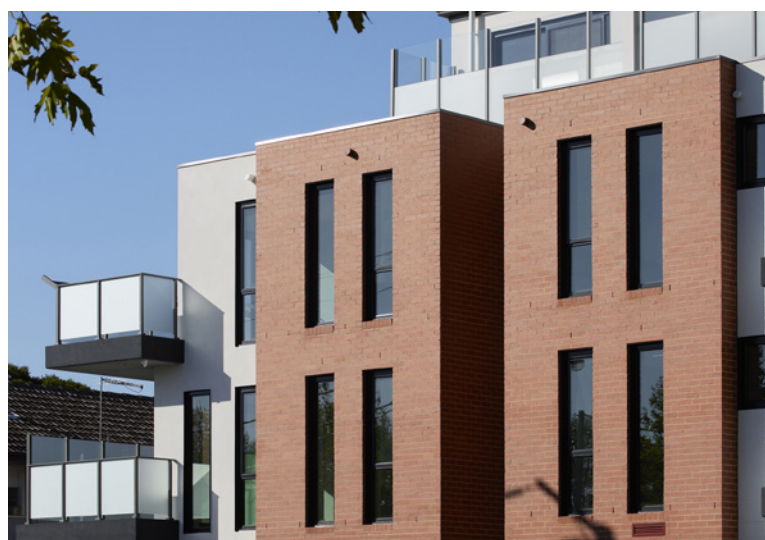
Unison Fairfield by Foreground Architecture for Unison Housing, a recently completed age friendly social housing development.
